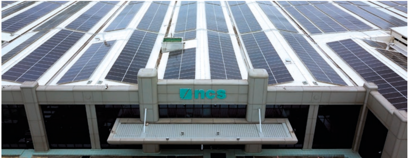
NCS Bedok Data Centre, one of the largest single-roof solar-powered data centres in Southeast Asia
